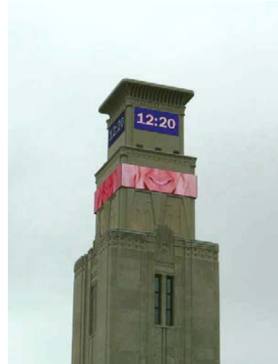
Akron Beacon Journal, 25' tall by 13' wide Fiberglass Tower replicating Indiana Limestone.
