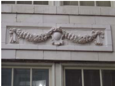
West Technical High School Restoration, Decorative fiberglass scroll elements.
