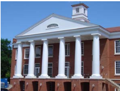
Western Reserve Academy, Hudson OH, 48" dia by 28' fiberglass columns.
