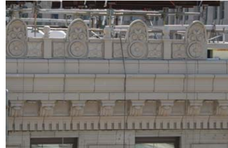
Terminal Tower 15th floor, 10' tall fiberglass cornice replacing terra cotta cornice.
