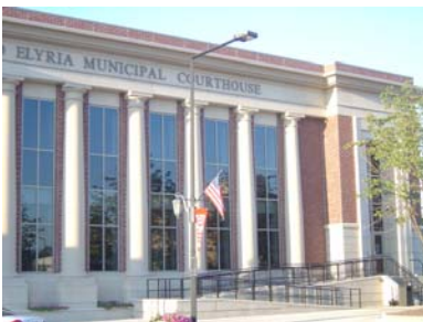
Elyria Municipal Courthouse, 40" dia columns and cornice replicating stone.
