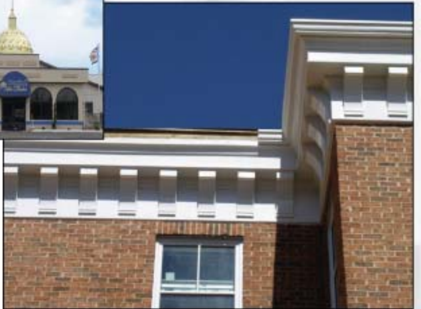
FRP Cornice and Brackets
