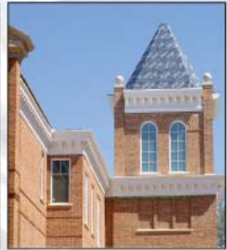
FRP Cornice and Brackets
